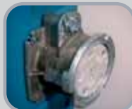
Prise interverrouillée 00 VCA 40 A 3 N+N+PE
